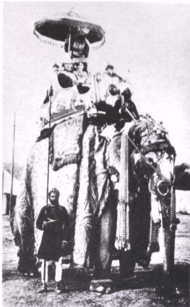
19 Curzon and Mary make their state entry into Delhi for the Coronation Durbar, 1903
